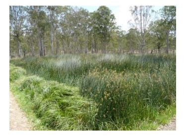
The Jubullum WWTP treats approximately 60 kL per day. Sewage is pre-treated by septic tanks from each household before entering an oxidation pond. The constructed wetland provided additional tertiary treatment following the oxidation pond before reuse within a citrus orchard. The constructed wetland consists of a 500 m<sup>2</sup> FWS wetland followed by a 300 m<sup>2</sup> HSSF wetland.
